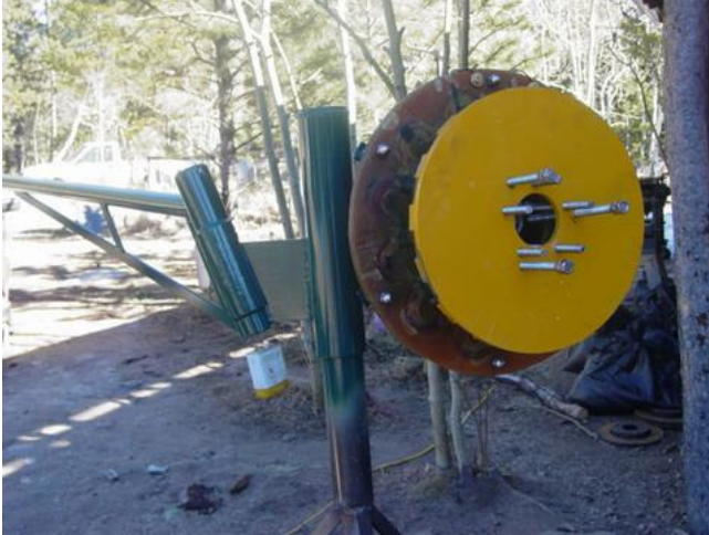
Second (Opposite) Rotor Being Lowered Into Position
